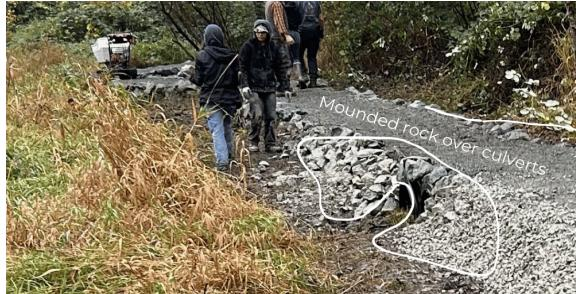
Description: Repairing and reinforcing the rock wall on the elevated trail. 4x8 will be delivered in piles, ballast rock will be delivered in buckets.
