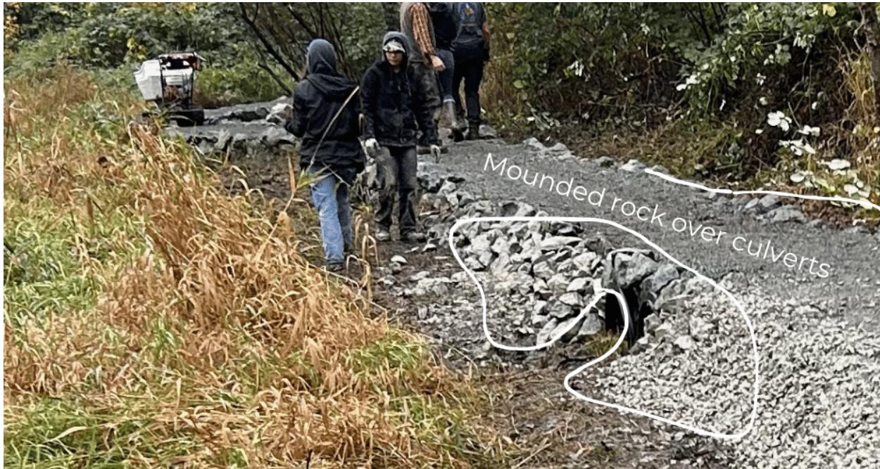
Description: Repairing and reinforcing the rock wall on the elevated trail. Rake up grass while we wait for first loads of rock to arrive. 4x8 will be delivered in piles, ballast rock will be delivered in buckets.
